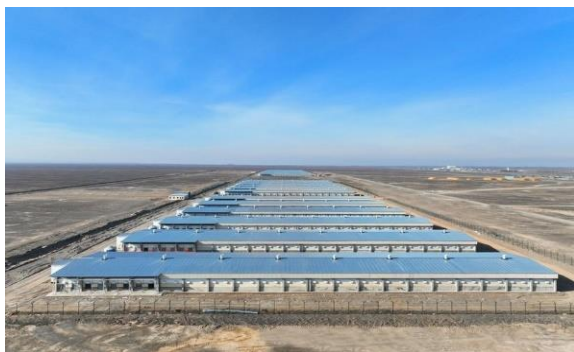
Figure 1 – General view of the production buildings of «PRIMA KUS» LLP
